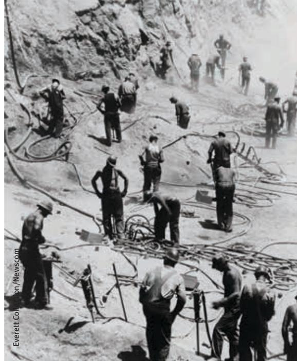
Before the dam could be built the Colorado River had to be diverted through tunnels. This piece of equipment, named a “jumbo rig,” was designed to speed up the tunnel drilling process. Built on the back of a 10-ton truck, 24 to 30 drills could be operated at once. Right: Drillers excavating the dam foundation on the Nevada side of Boulder Dam, 1933.
