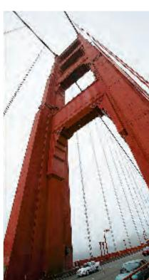
The Golden Gate Bridge – Opened in 1937 after four years of construction, the Golden Gate connects San Francisco and Marin County to the north. Its central span is 1,650 feet long and its Art Deco steel towers are 750 feet high. Each of the bridge's cables weighs more than 7,000 tons.
